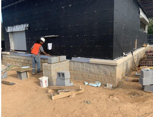
CSK- Concession Precast Installation
